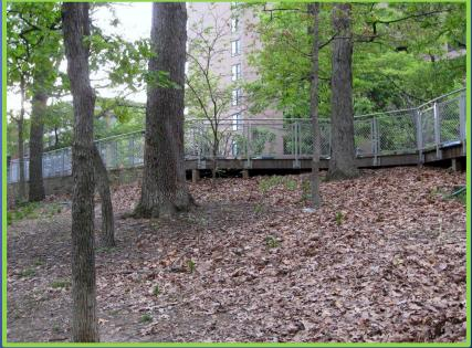
Wooden Boards Allow Rain to Pass Through – Reduces Water Run-off and Helps Prevent Debris from Accumulating and Decaying
