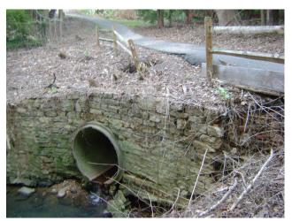
Stormwater from this outfall in Bluemont Park has eroded the surrounding wall and earth, undermining the fence and the pedestrian/bike path.
