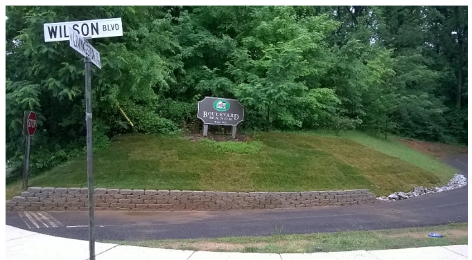
Upton Hill Regional Park planted grass and constructed a retaining wall, improving our neighborhood's northwest entrance.
